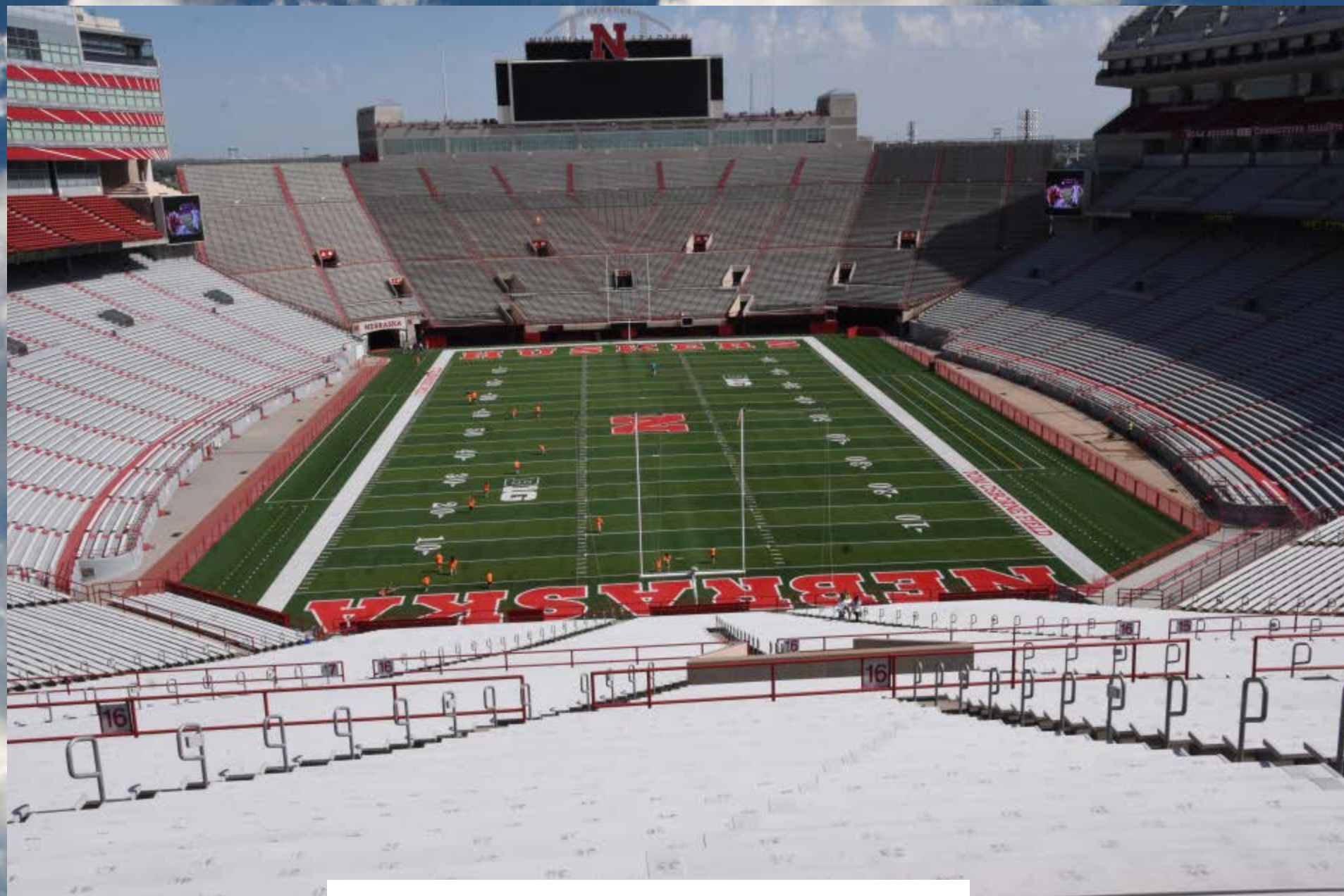
At the top of the South Stadium
